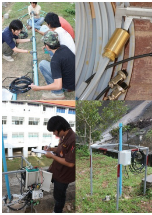
Figure 10: Instrument installation and monitoring.
