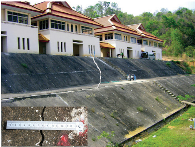
Figure 2: Studied slope and crack observed on concrete face.
